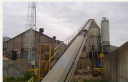
Picture (1): Snapshot of the batch plant
