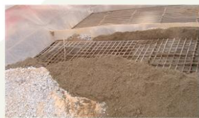
Picture (6): The Ground hopper to receive gravel and sand
