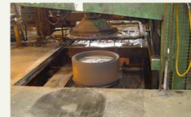
Picture (20): The core comes up to make the manhole visible
