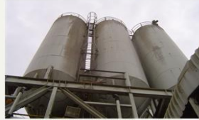
Picture (2): The main silo with five partitions
